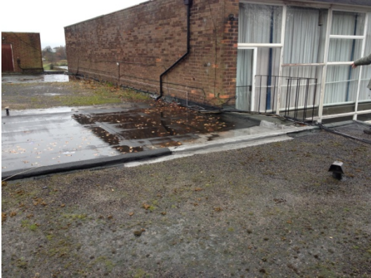
Roof Patch Repairs, roof area 3.
